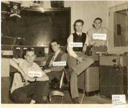
WJBO Control Room
