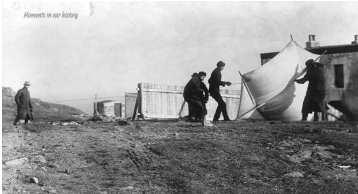
Preparing the kite known as Marconi kite, which supported the receiving aerial for reception of the first transatlantic telegraph signals, at St John's, Newfoundland. Guglielmo Marconi, the Italian physicist and inventor can be seen on the extreme left. 12th December 1901
